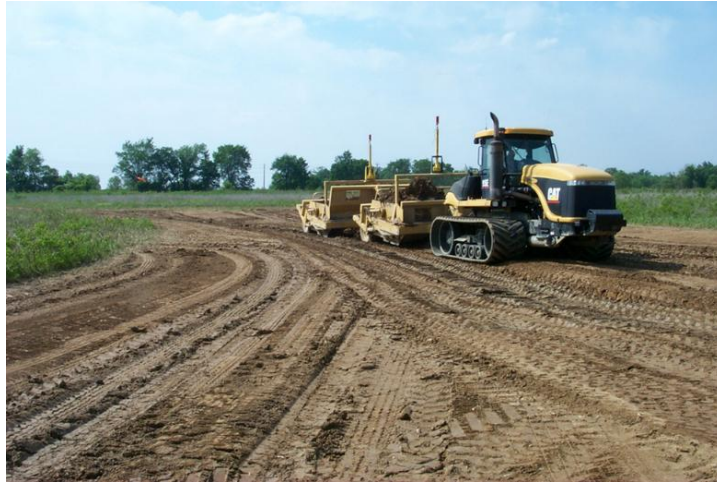
Figure 4. Land-forming a former agricultural site to restore topographic relief that was removed when the site was under cultivation (Photo credits: USDA, NRCS).
