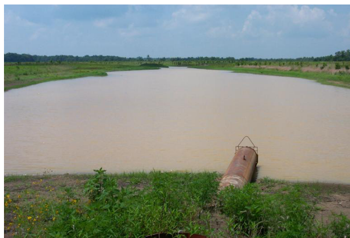
Figure 5. Water control structure installed to manage water retention and wetland functions within a shallow depression on an afforestation site. Notice the saplings established in the right background where the topography grades to a higher elevation (Photo credit USDA, NRCS).
